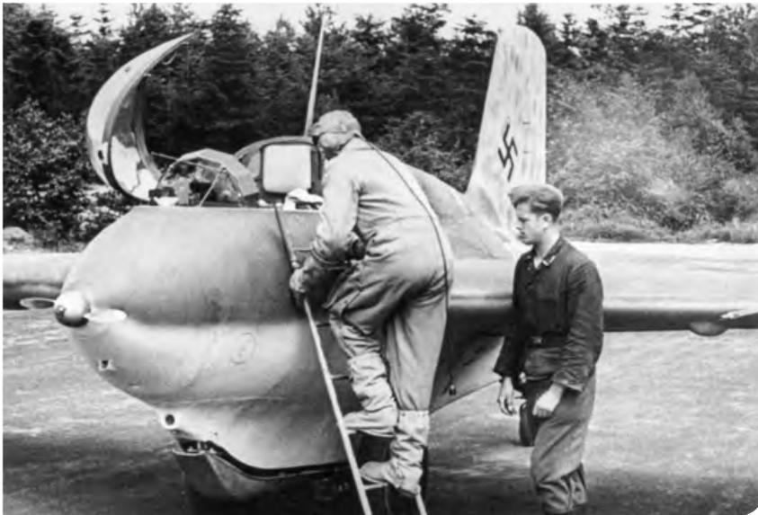
The walls of the two fuel tanks to the left and right of the pilot were made of very thin metal. In a hard landing, the remnants of the highly corrosive fuel often leaked.
